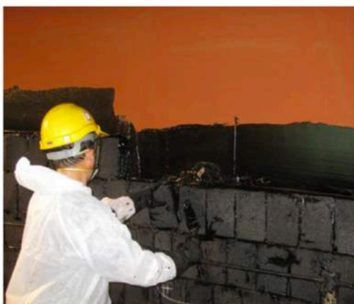
Picture 4: Pennguard lining installation
