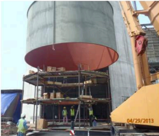
Picture 2: Steel can ready for positioning into the chimney
