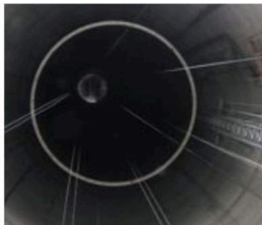
Picture 5: Pennguard lining completed in the vertical part of the steel flue
